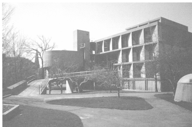
Fig. 12. Carpenter Center, Harvard University, Cambridge, MA. Le Corbusier. Angled brise soleil admit direct winter sun and reflected sunlight year-round.
